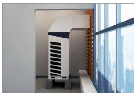
Installation of duct
